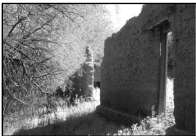
Munguia Homestead prior to brush removal. Photo by J. Dale 2005
